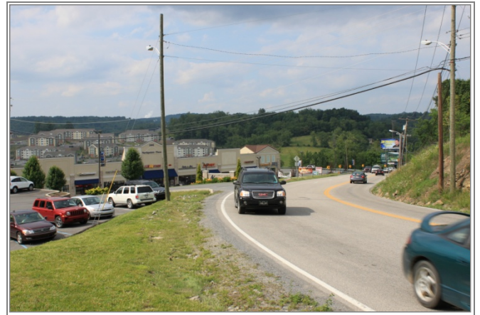
Figure 3. Three-Lane Section with Climbing Lane
