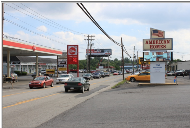
Figure 2. Three-Lane Section with Left-Turn Lane
